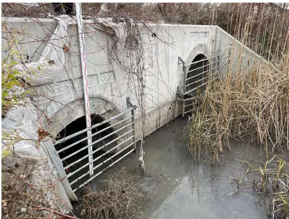
Photo A.2: Markham Road Culvert System Outlet
