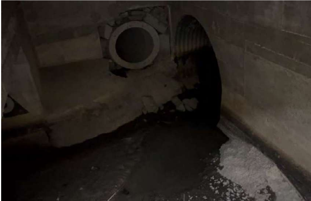
Photo A.3: Markham Road Culvert System 1500 mm Diameter CSP
