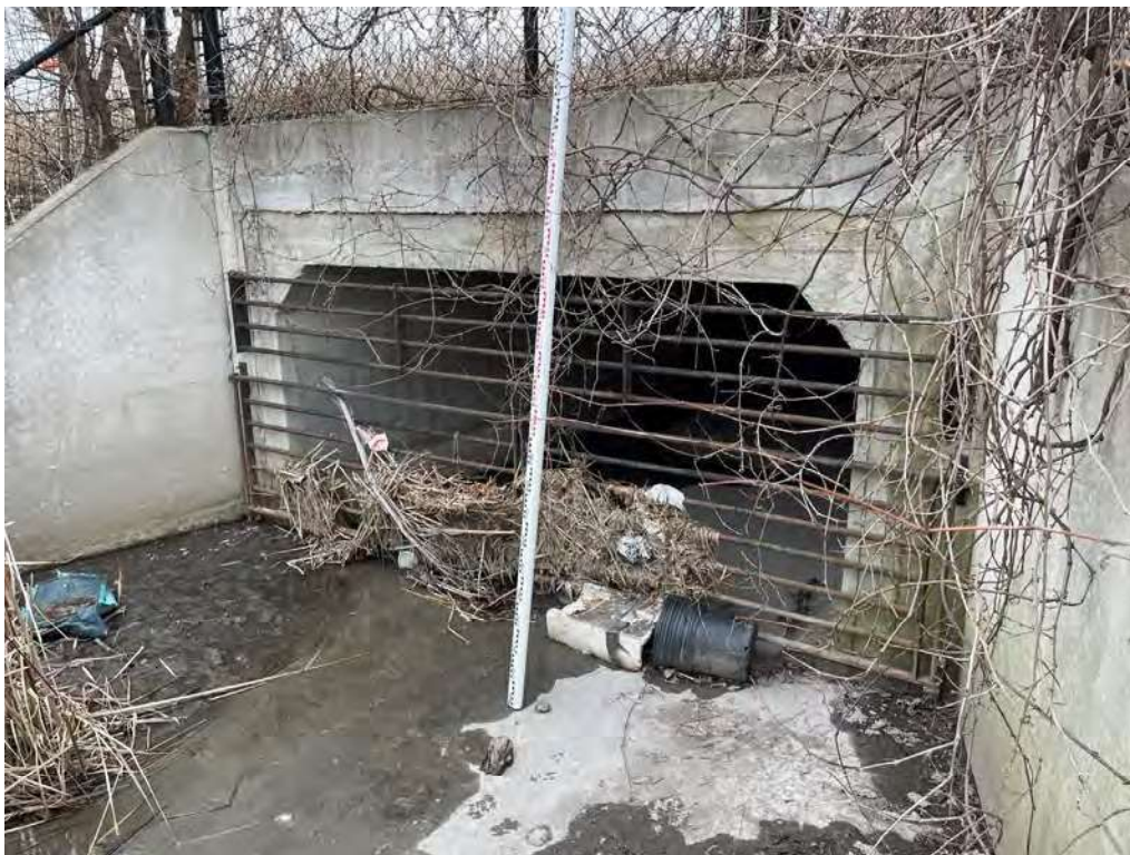
Photo A.1: Markham Road Culvert System Inlet
