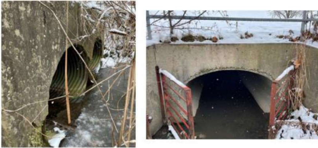
Figure 14 – Upstream Face (Left) and Downstream Face (Right)
