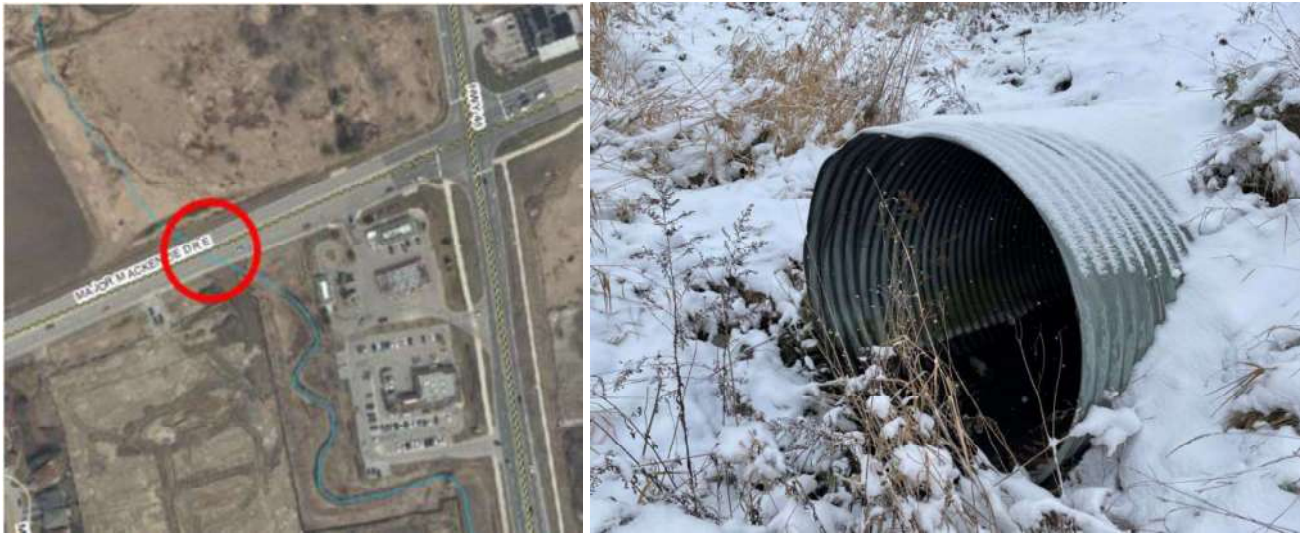
Figure 10 – Crossing Location (Left) and Site Photo (Right)
