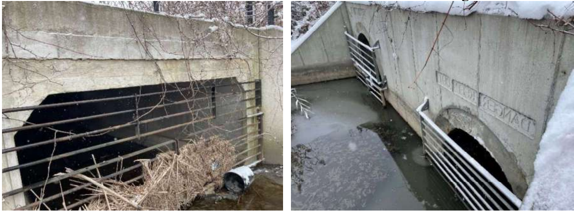
Figure 12 – Upstream Face (Left) and Downstream Face (Right)
