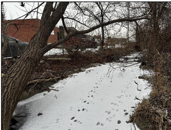
Figure 3-6: Looking upstream at channel in close proximity to parking lot
