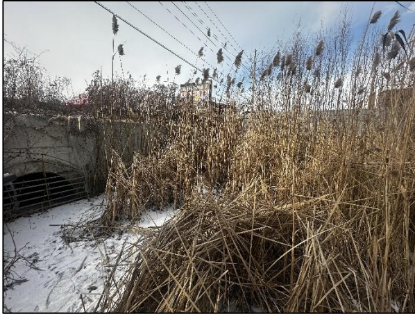
Figure 3-10: Looking upstream at the twin culvert with concrete headwall and the start of Phragmites within the reach
