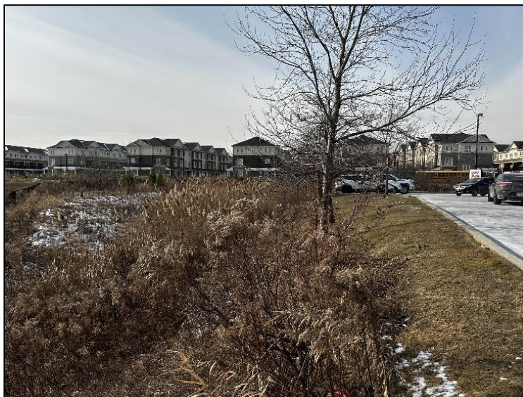
Figure 3-30: Phragmites infilled channel adjacent to commercial properties and parking lot leading to increased drainage and run-off into the channel and the outfall
