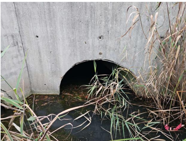
Figure 2-4: Major Mackenzie Drive East Downstream Culvert Face
