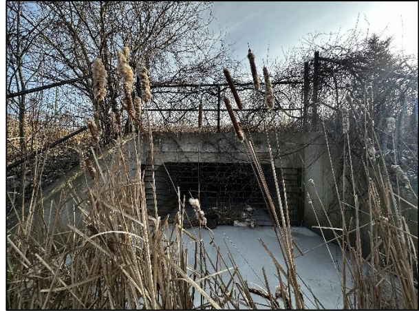
Figure 3-17: Concrete box culvert located at the downstream extent of the reach at Markham Road
