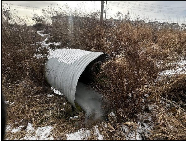
Figure 3-18: Looking at the CSP culvert upstream of Major Mackenzie Drive East conveying flow from open agricultural land
