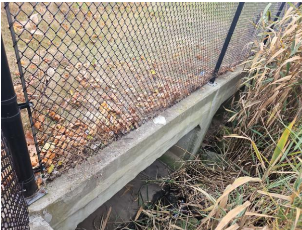
Figure 2-14: Bur Oak Avenue Upstream Culvert Face
