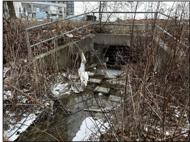
Figure 3-9: Anderson Ave culvert at upstream extent of the reach
