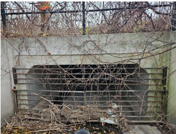
Figure 2-6: Harvard Way Upstream Culvert Face
