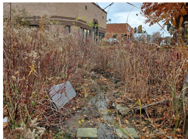
Figure 2-13: Downstream Channel (Near Anderson Avenue)
