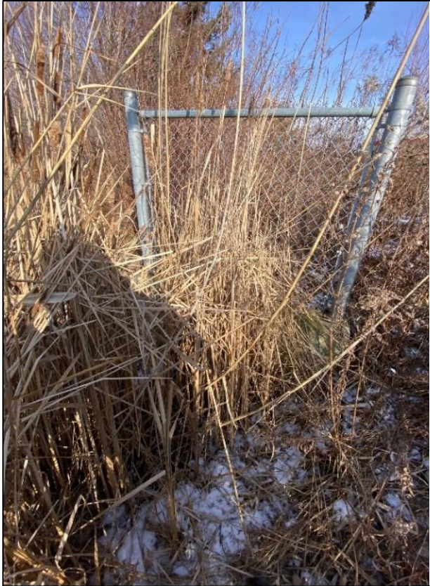
Figure 3-28: Looking directly at the buried stormwater outfall with concrete headwall and fence
