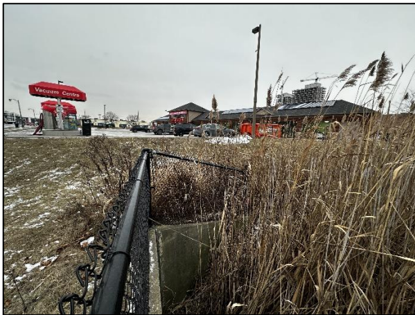
Figure 3-4: Upstream side of Bur Oak Ave culvert, facing west towards Carwash
