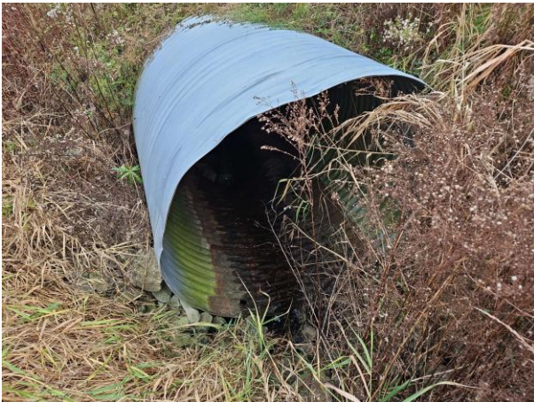
Figure 2-2: Major Mackenzie Drive East Upstream Culvert Face
