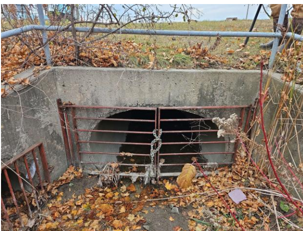
Figure 2-12: Downstream Culvert Face (Near Anderson Avenue)
