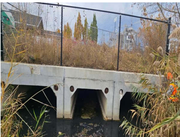
Figure 2-16: Bur Oak Avenue Downstream Culvert Face
