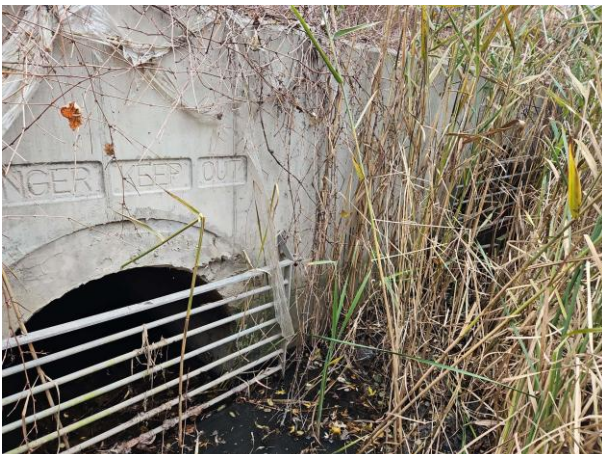
Figure 2-8: Markham Road Downstream Culvert Face
