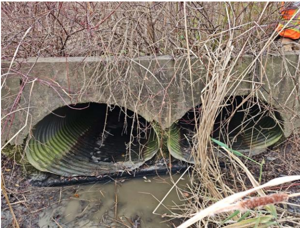
Figure 2-10: Upstream Culvert Face (Near Anderson Avenue)
