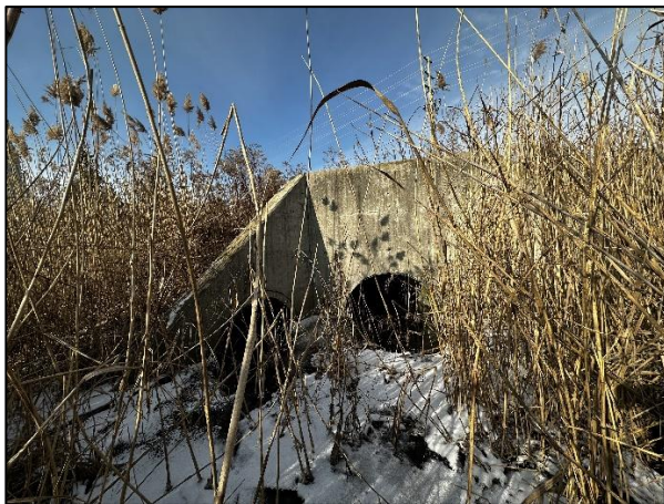
Figure 3-14: CSP culvert with concrete headwall located at upstream extent of reach conveying flow under Major Mackenzie Road East
