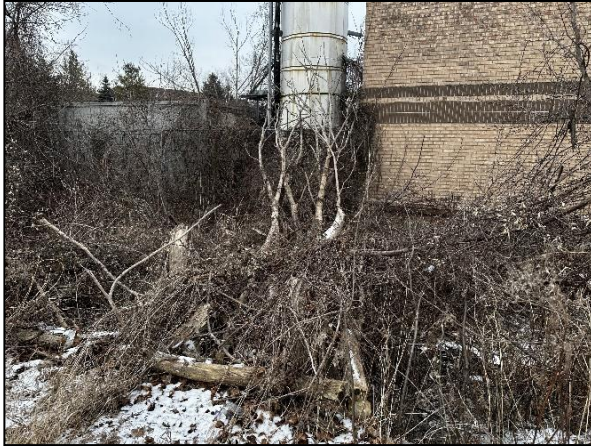
Figure 3-22: Severe debris jam approx. 115 m downstream of Anderson Ave culvert
